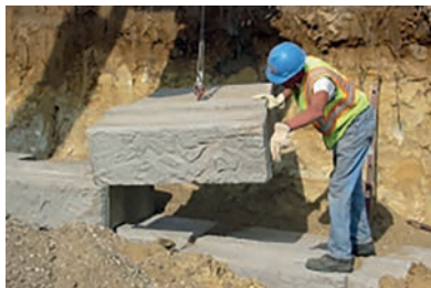
Position layers, self-supporting retaining wall
