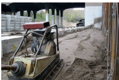
Backfill and compact
