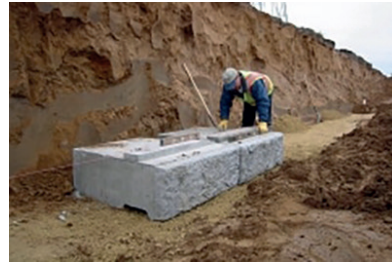
Position and level the base blocks
