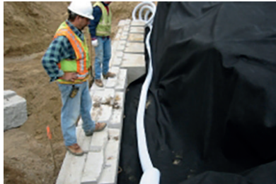
Position filter fabric
