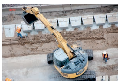
Add extra layers for self-supporting retaining wall
