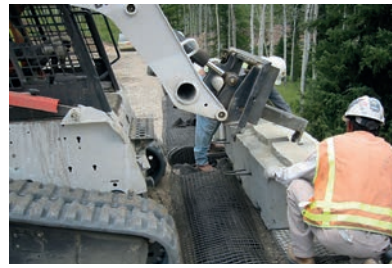
Add extra layers for geogrid retaining wall
