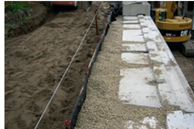
Position drainage materials
