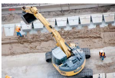
Add extra layers for self-supporting retaining wall
