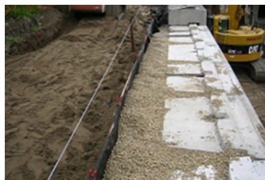
Position drainage materials
