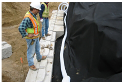
Position filter fabric
