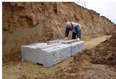
Position and level the base blocks
