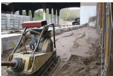
Backfill and compact
