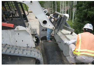
Add extra layers for geogrid retaining wall
