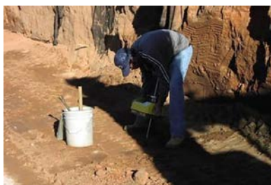
Check compaction regularly
