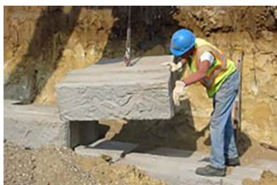
Position layers, self-supporting retaining wall
